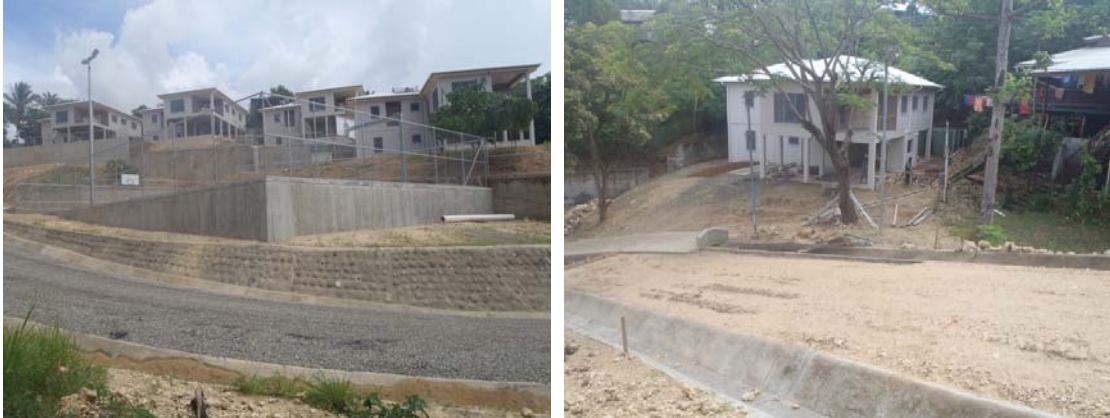
Figure 2.0: After with Completed Building & Site Works.
